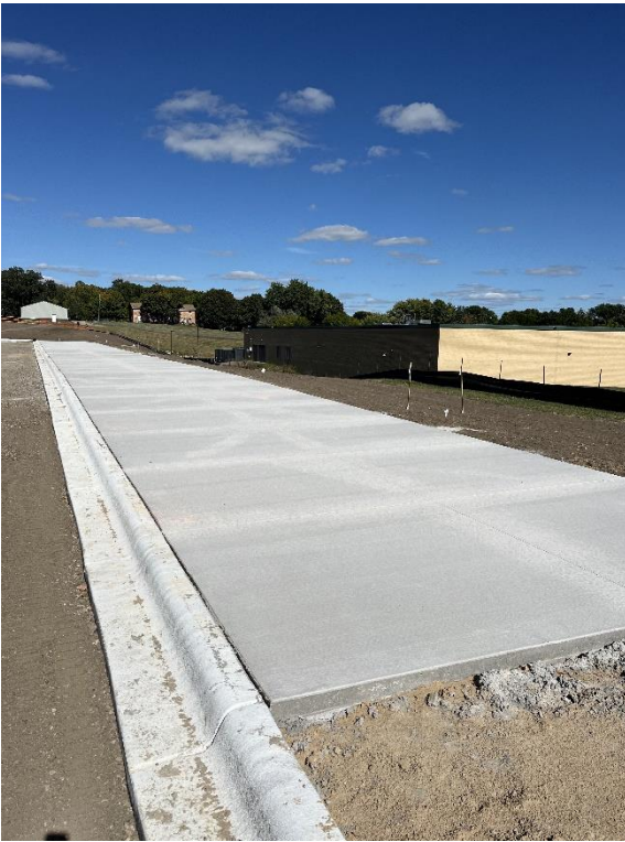
Concrete walk poured for bus drop-off area
