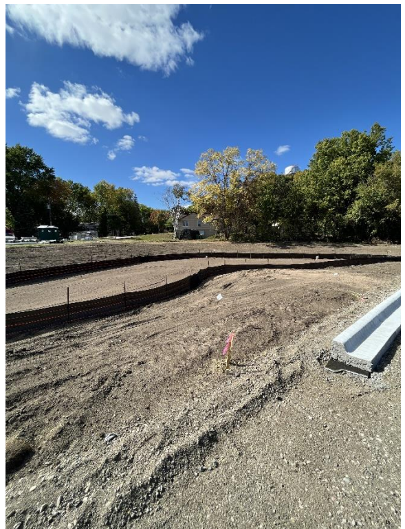
Retention basin subgrade complete along with drain tile installation
