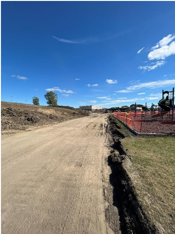
Removal of top soil complete at entry to new bus loop
