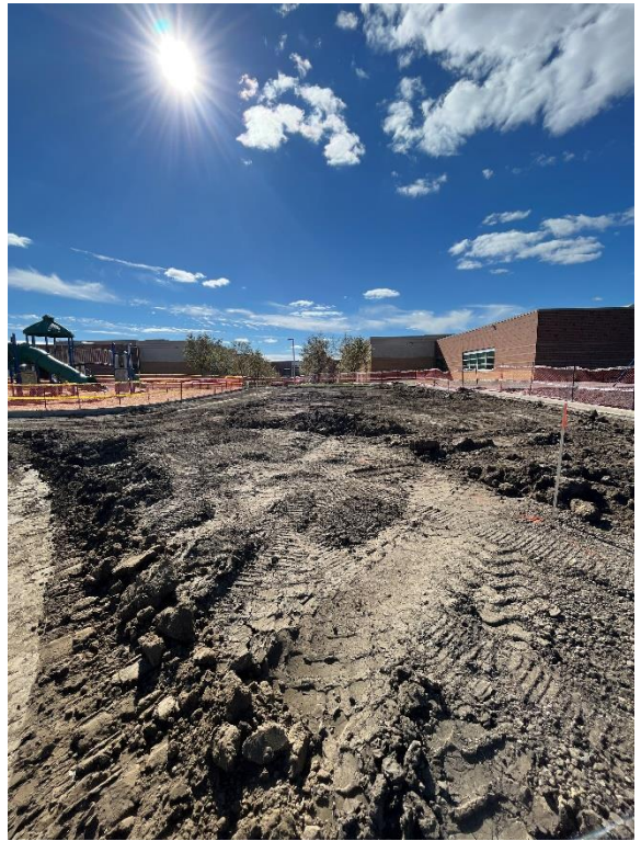
Removal of old asphalt complete between playgrounds
