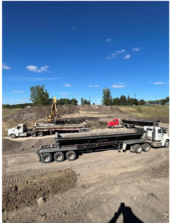
Excavation and exporting of unusable common soils underway
