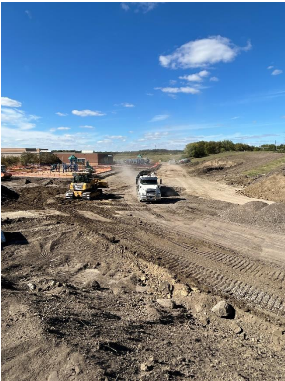
Stripping of topsoils complete at Southern end of new bus loop
