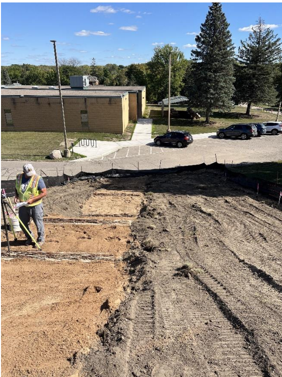
Concrete stairwell surveying and preparing for pouring of stairs
