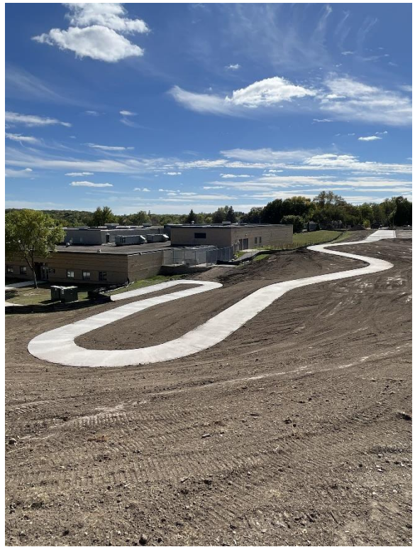
Entirety of ADA concrete path complete and remainder of site brought to finish grade
