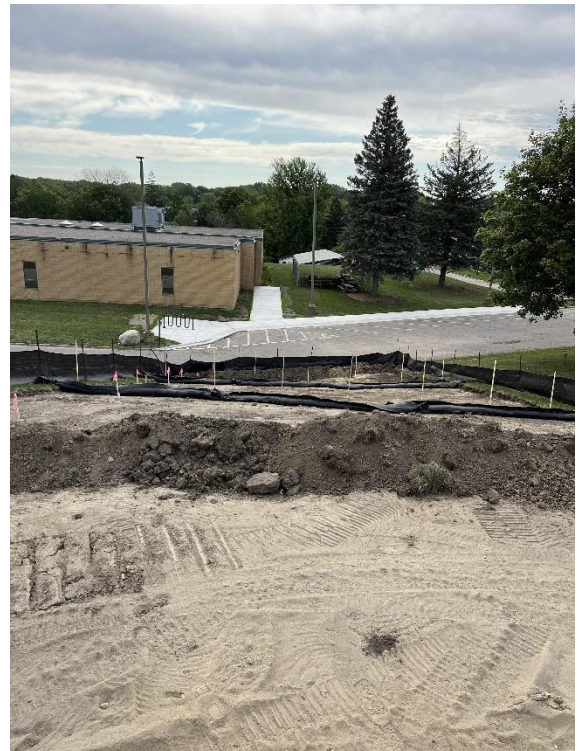
Top soil removed for new stairwell leading to South entry
