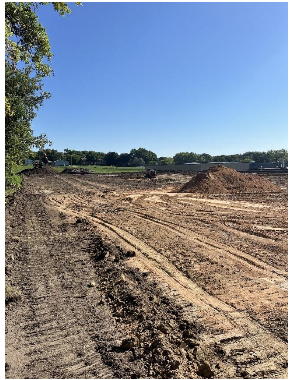
Stripping of topsoil and ag lime from youth field for MS bus loop
