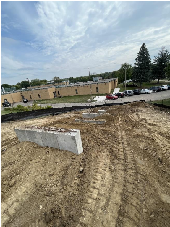
Concrete stair footings and foundation walls poured and backfilled
