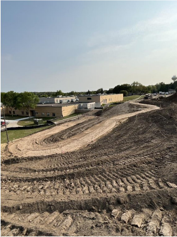
ADA path grading underway, preparing for concrete
