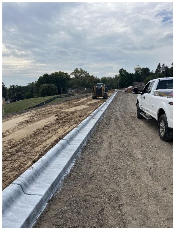
Curb and gutter surrounding site installed and backfill for concrete walks underway
