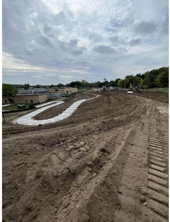
ADA path concrete pour underway, remainder of path to be poured Monday
